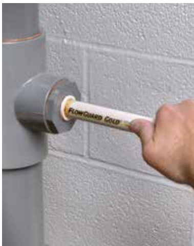
Installation of C-PVC pipes
